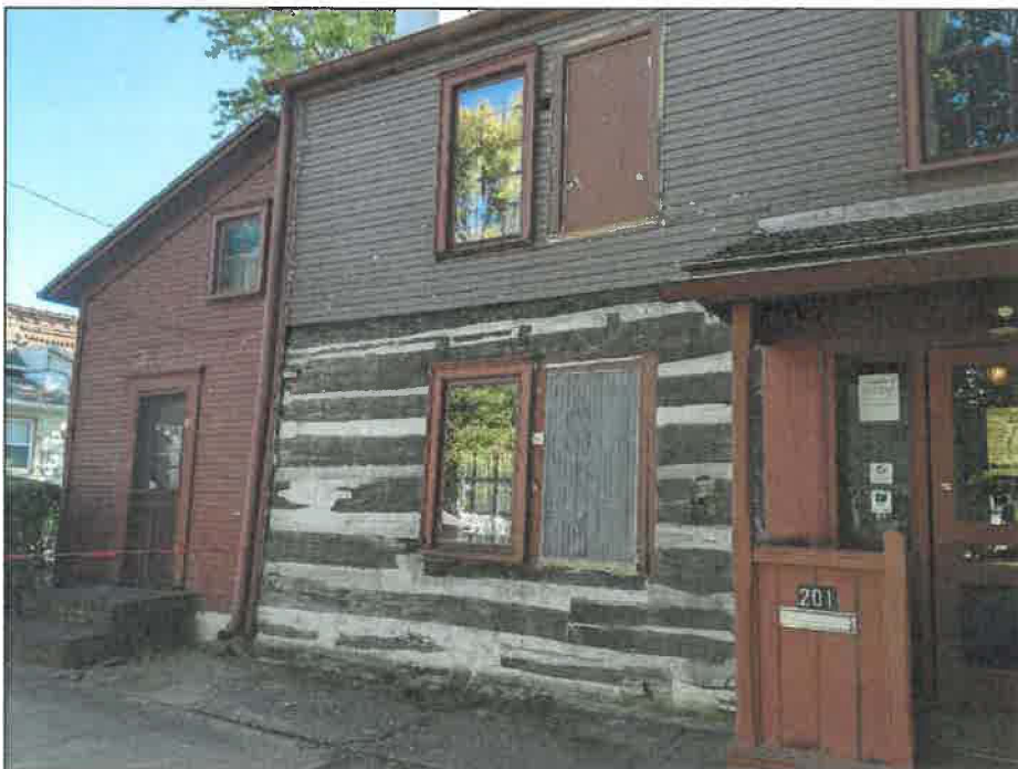
Detail of the west elevation, facing Mulberry Street, after removal of the siding.
