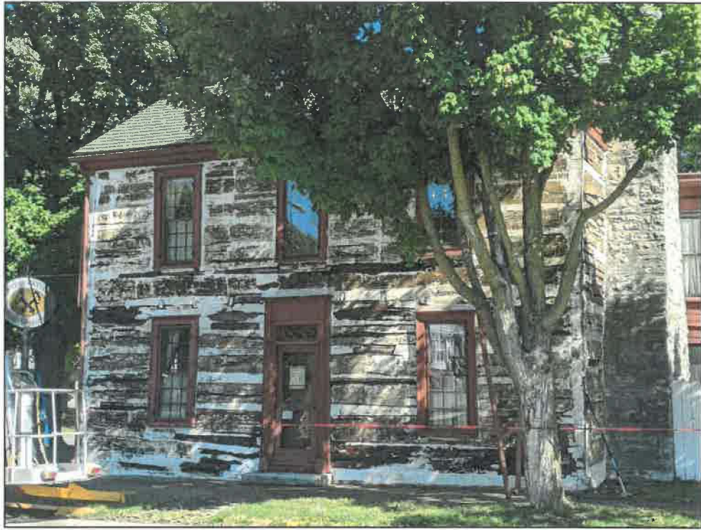
Overview of the south elevation, facing Water Street, after paint removal.
