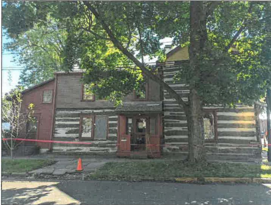
Overview of the west elevation, facing Mulberry Street, after removal of the siding.
